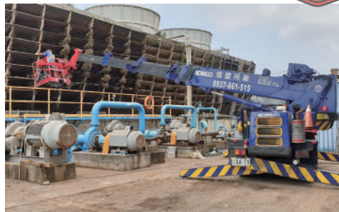
Protection for elevated work activities
