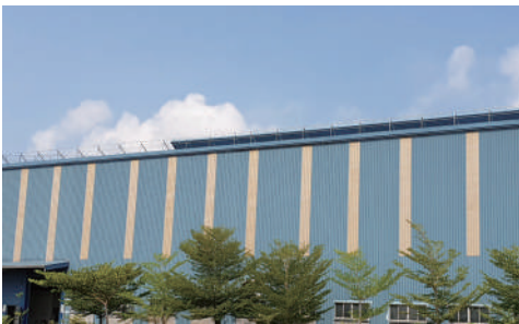
Installation of new protective rails around the rooftop
