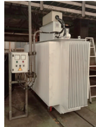
Replaced APL No. 4 electrolytic rectifier transformer Replacement of outdated equipment
