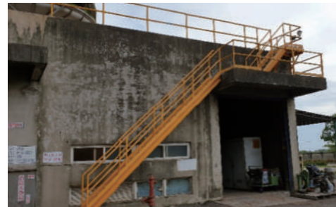
Outdoor ladders replaced with stairs
