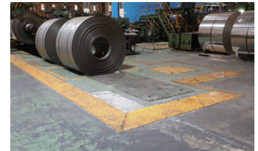
Ground leveling work
