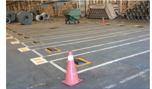
Implementation of controls for steel coil storage
